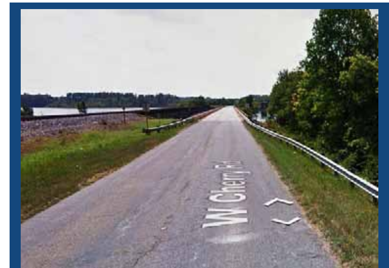
Figure 5-14. Causeway and Bridge Over Lake Hartwell
